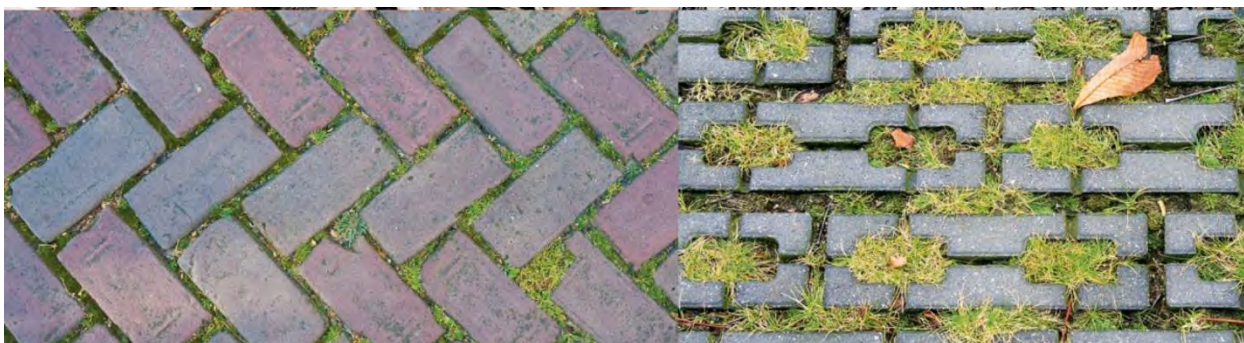
Figure 8: Water Permeable Pavements
