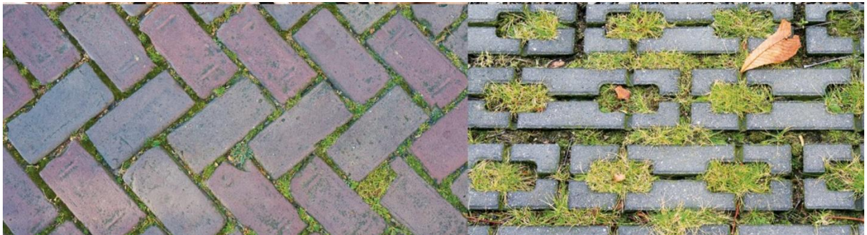
Figure 8: Water Permeable Pavements
