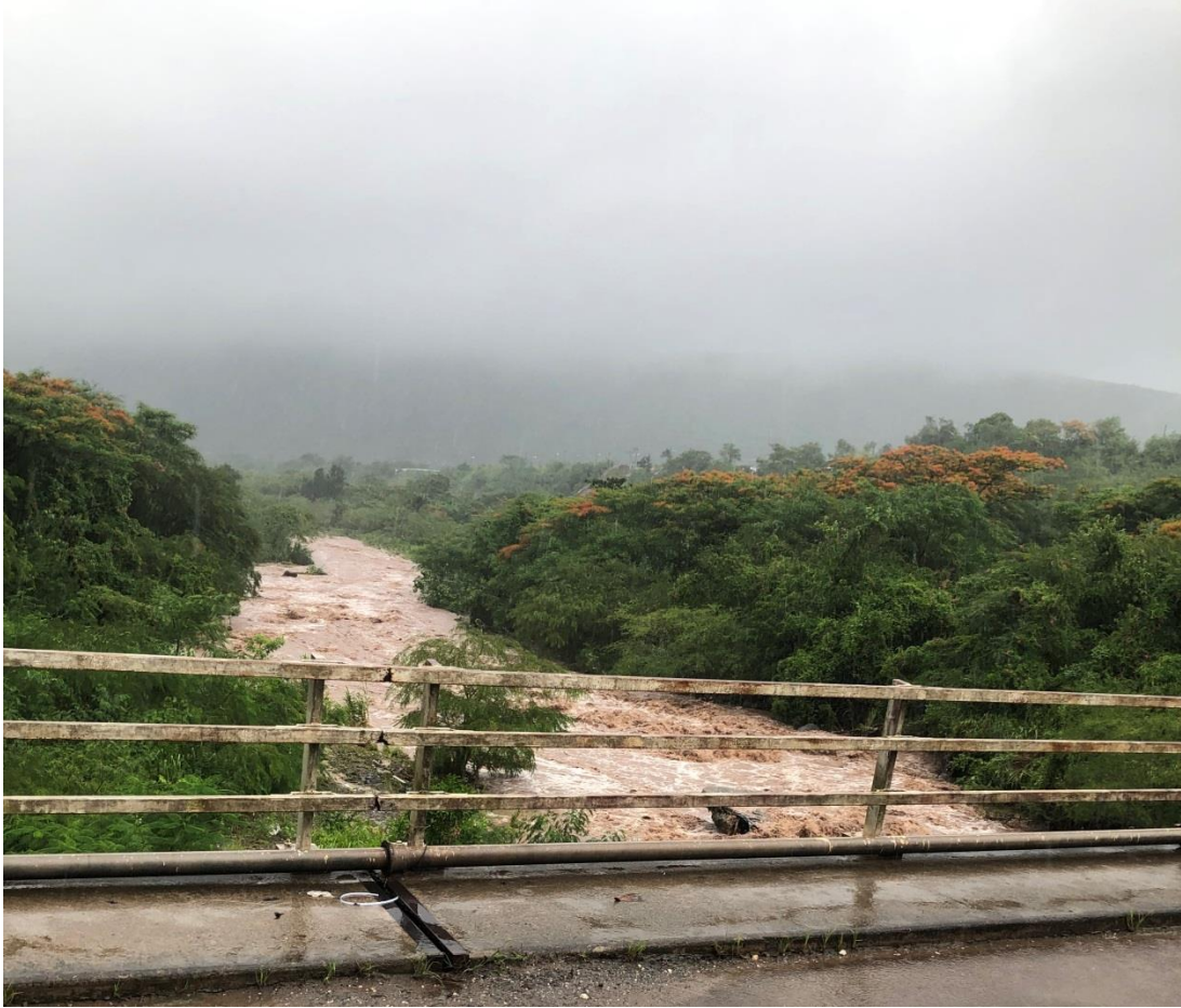
Figure 5-12: Hope River in spate viewed from Kintyre Bridge April 20, 2022.
