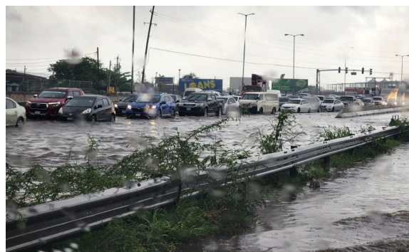
Figure 1.1: Flooded section of Marcus Garvey Drive following heavy rainfall event on Thursday, June 8, 2023. (Our Today, 2024)
